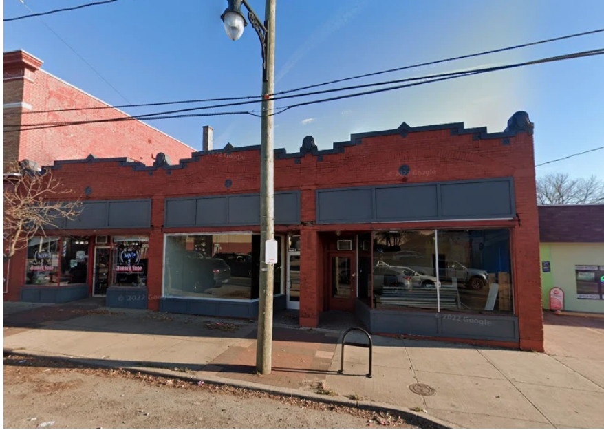
Lopez plans to add two stories to the existing building. Credit: Google Street View
